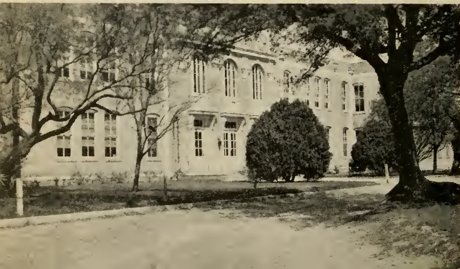
Faith Hall Holding Institute, Laredo, Texas
